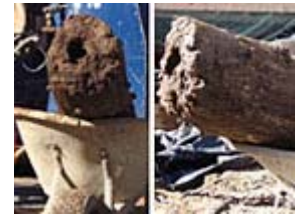
A section of the 19th century water main
